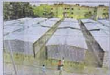
Temporary stalls that will be handed over to shop-keepers on April 19. Pictures by Sarat Kumar Sinha
